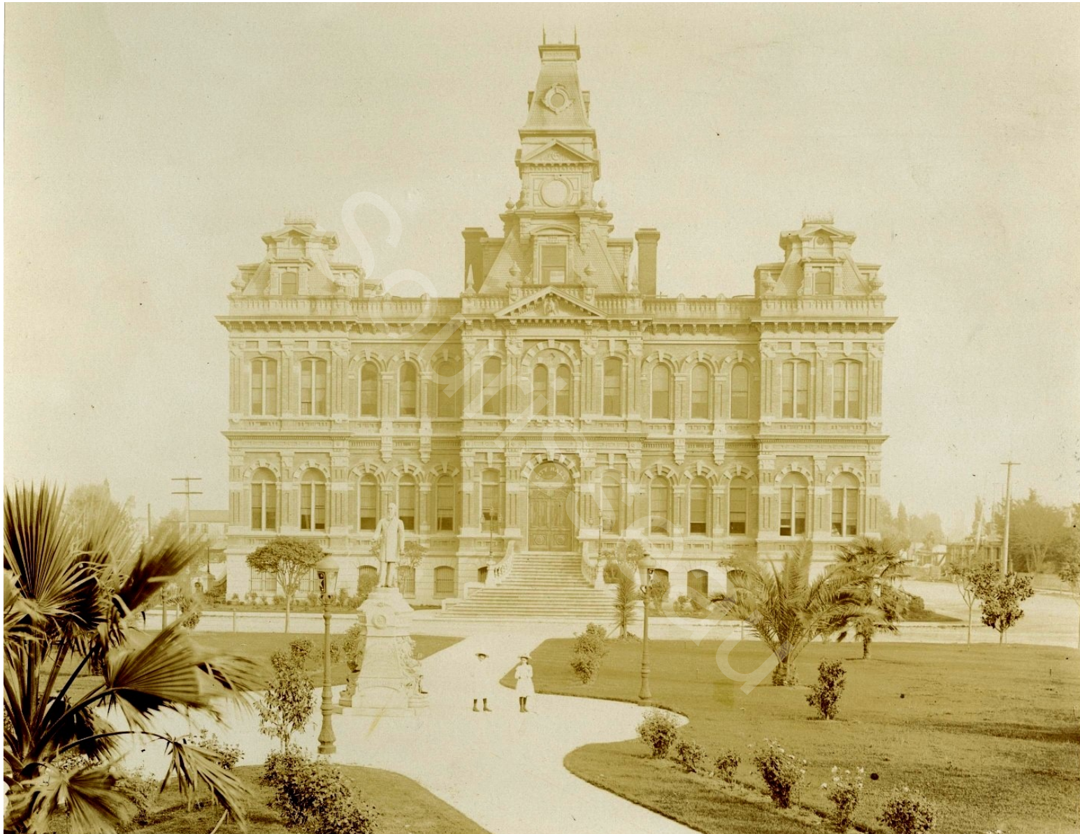
[122] Lenzen Designed San Jose City Hall. If there is one building that captures the status and vitality of urban San Jose in the late Victorian era, it is the 1889 City Hall. Designed by Theodore Lenzen, the architecture reflects its era. The mansard roof displays the latest European style in civic grandeur and stone facings show its substantive budget. Lenzen felt using sandstone was an extravagance, but civic leaders pointed out that other local cities had made liberal use of stone from San Jose's Goodrich quarry and San Jose deserved the best.
