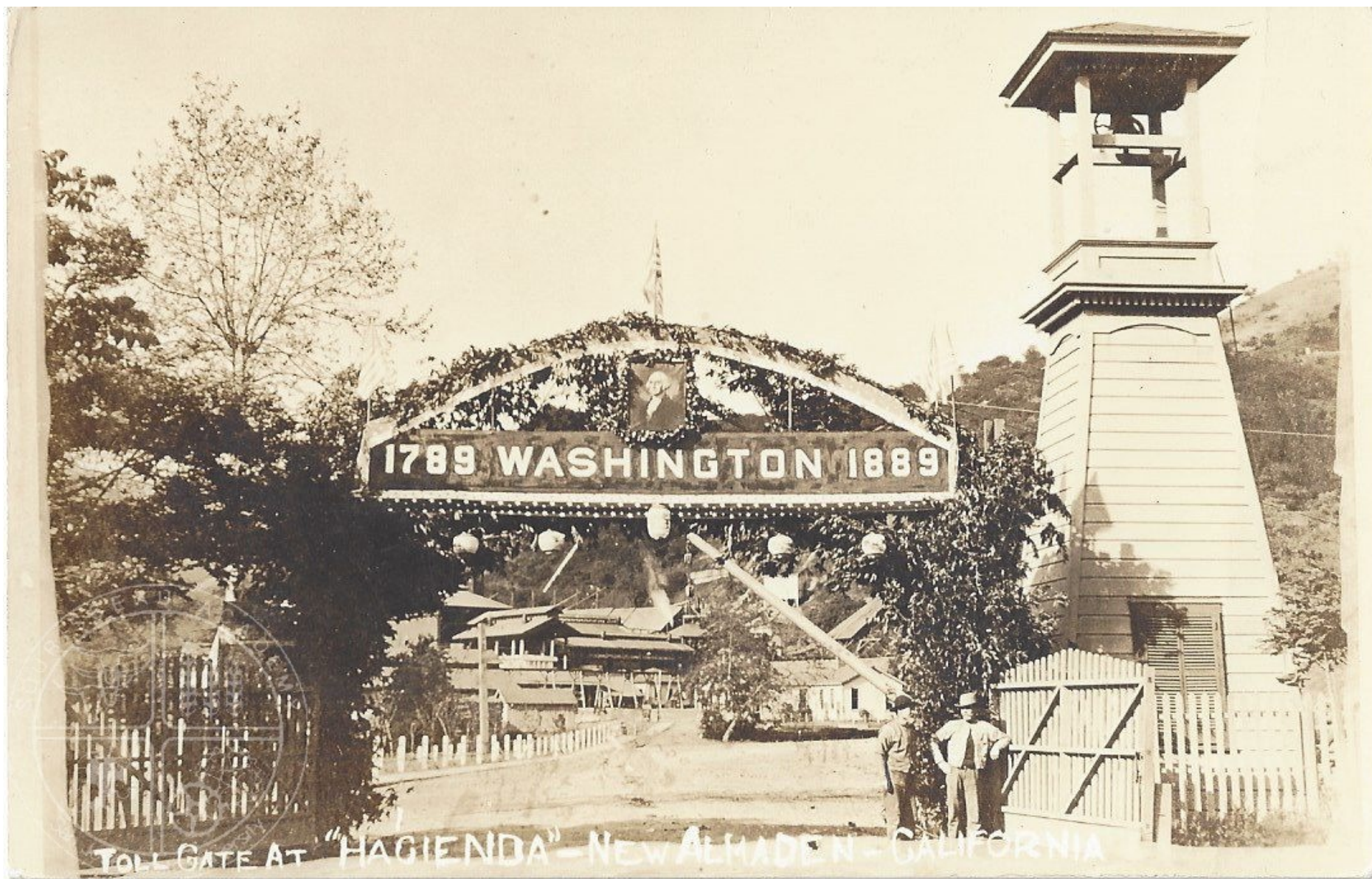
[76] New Almaden celebrates our first President - In 1889, the citizens of New Almaden's Hacienda celebrated the centennial of George Washington's presidency. This decorated gateway — a toll gate — led to the Quicksilver Mining Company's business offices and industrial buildings.
