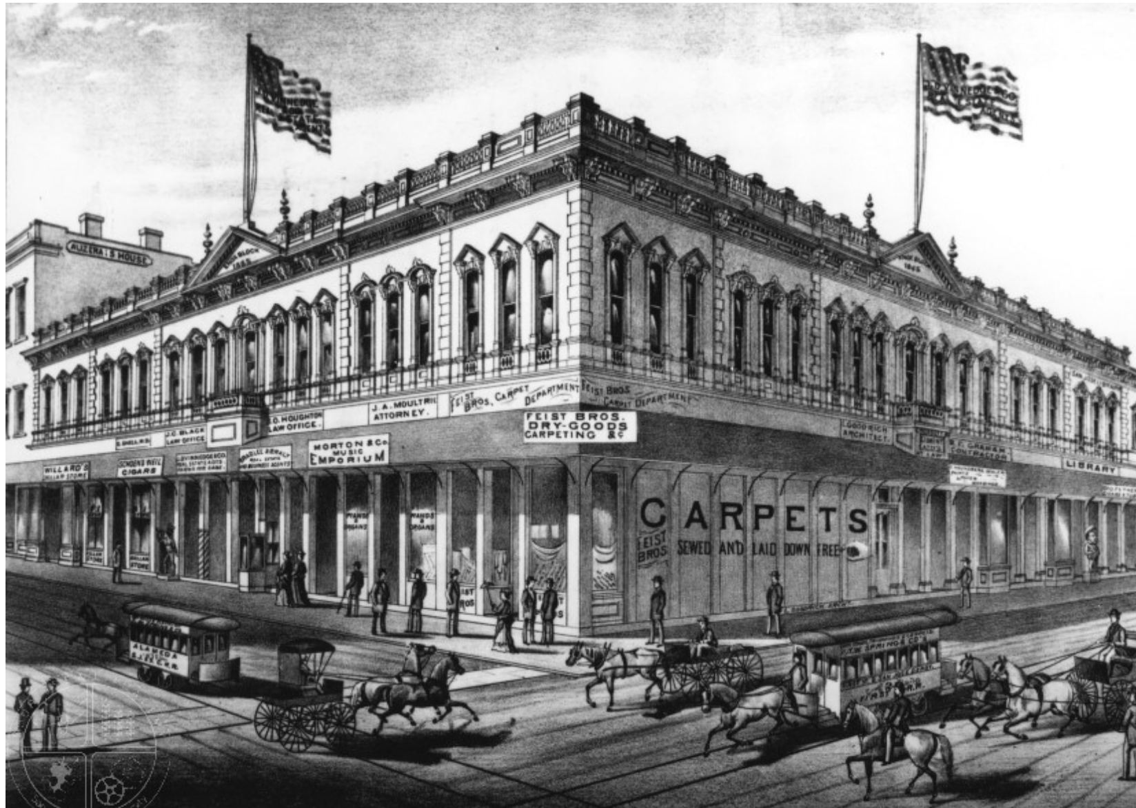
[1] Knox & Beans Bank. In 1865, after making a fortune in hydraulic mining on the South Yuba River, Dr. William J. Knox moved to San José and built the Knox Block. Located on the northwest corner of First and Santa Clara Streets, the Knox Block served as San José's principal office building for many years. In 1866, Knox and his brother-in-law T. Ellard Beans established the Knox & Beans Bank, San José's first, in the Knox Block. Reorganized and incorporated as the Bank of San José in 1868, the bank remained here until 1872 when it moved into its new three-story building directly across First Street. The Knox Block was demolished in 1945 and replaced by the J. C. Penney's department store.
