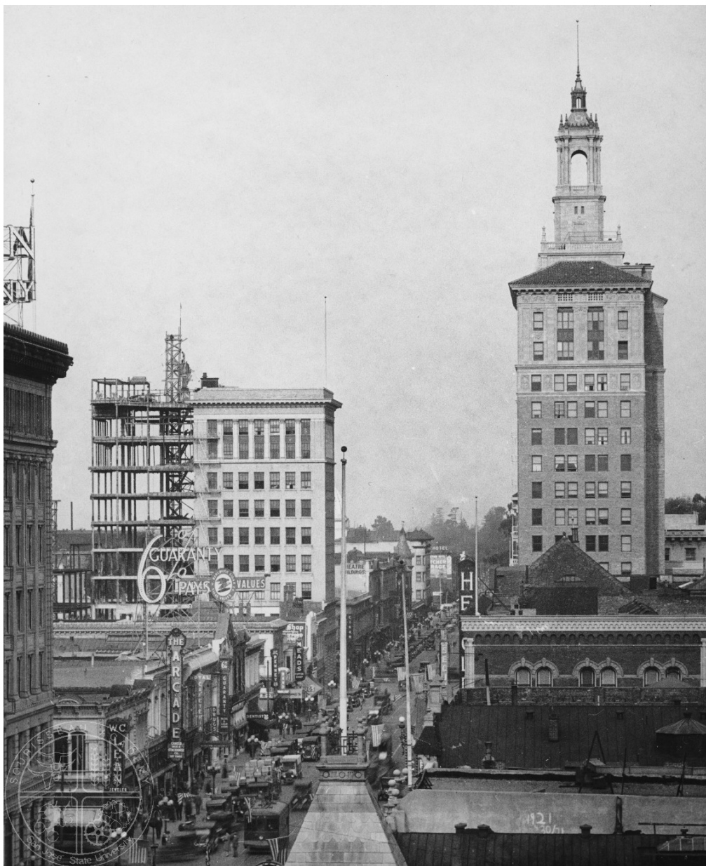
[16] South First Street 1927. Looking north on South First Street in 1927, a portion of the Garden City Bank is seen along the left edge of the image. In the background on the left, the First National Bank's addition is under construction on the former site of the San José Savings Bank. On the right is the recently completed Bank of Italy tower, which became the main San José office of the Bank of America in 1930, and still exists substantially unchanged externally.
