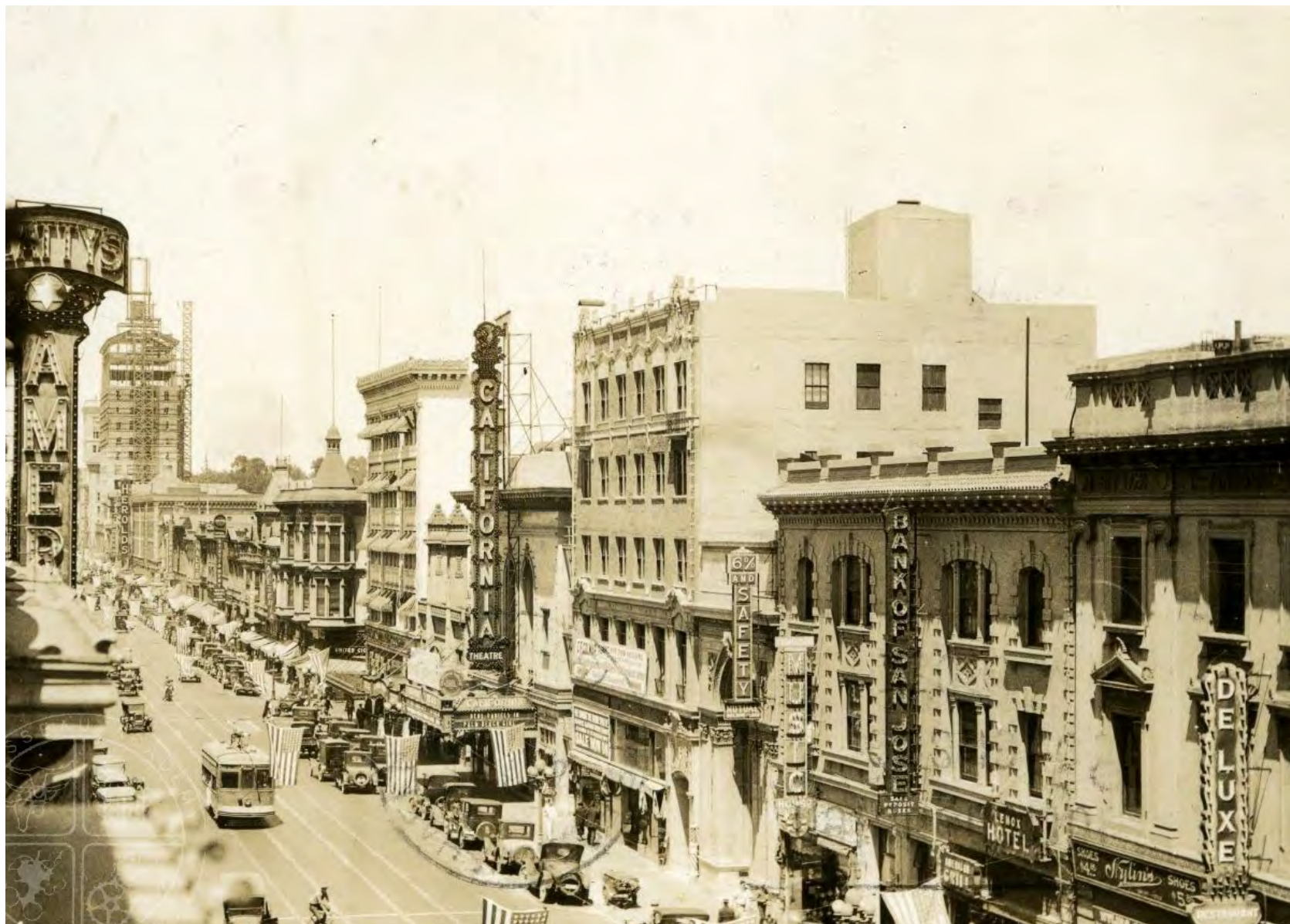
[14] South First Street 1926. Looking north on South First Street in 1926, the Bank of Italy tower is seen under construction in the background, and in the foreground the new first branch of the Bank of San José is seen in the city's theater district. The Bank of San José branch and the De Luxe Theatre were located where the U.S. District Court now stands. As buses came into service, San José's extensive street rail grid was abandoned by 1938, and the tracks torn up. The light rail tracks now running along First Street were replaced at great expense in the 1980s.
