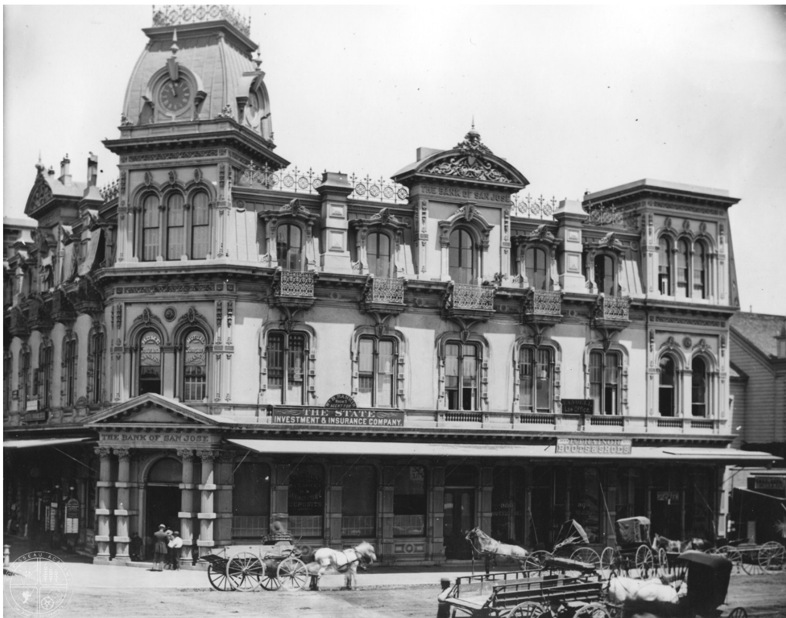
[2] 1872 Bank of San José Block. This building on the northeast corner of First and Santa Clara Streets, completed in early 1872, was the office of the Bank of San José until it was severely damaged in the great earthquake of April 1906. The clock tower, facing in four directions and visible from blocks away, was a San José landmark for many years. T. Ellard Beans, who served as its president from 1871 until his death in 1905, was succeeded by his son, William Knox Beans.
