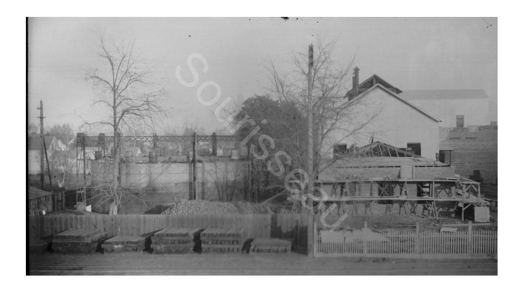
[23] **San Jose Gas Company.** The left half of this San Jose Gas Company panorama shows the massive expansion storage tank (the tank top moved up and down according to the amount of gas inside). Note the barrels on top of the tank — probably containing water for fire suppression.
