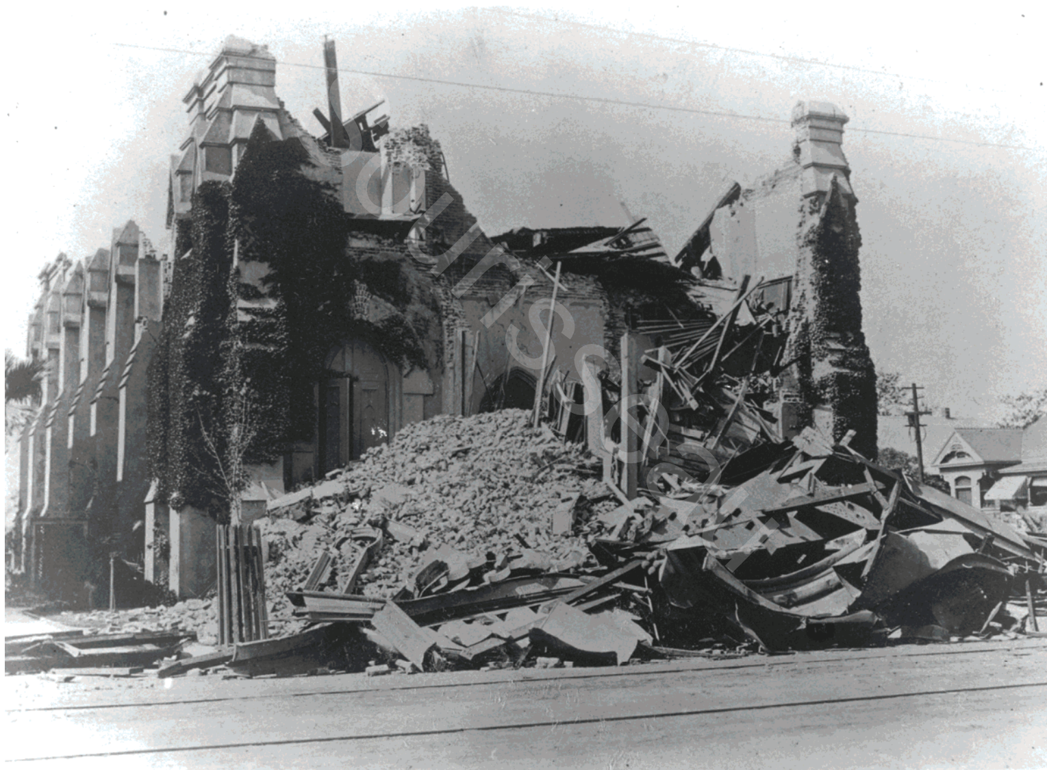
[39] St. Patrick's Roman Catholic Church, located at the northwest corner of Santa Clara and Ninth Streets, clearly suffered extensive damage in the quake. The tower and front wall fell across Santa Clara Street, and while the choir gallery remained intact, it was heaped with debris from the fallen roof. Additionally, the rear wall fell inward while the east wall fell outward. Undaunted by the destruction, parishioners set about rebuilding on the same site. The new church, completed in less than a year, served its parish for sixty-seven years, when a more modern structure replaced it.
